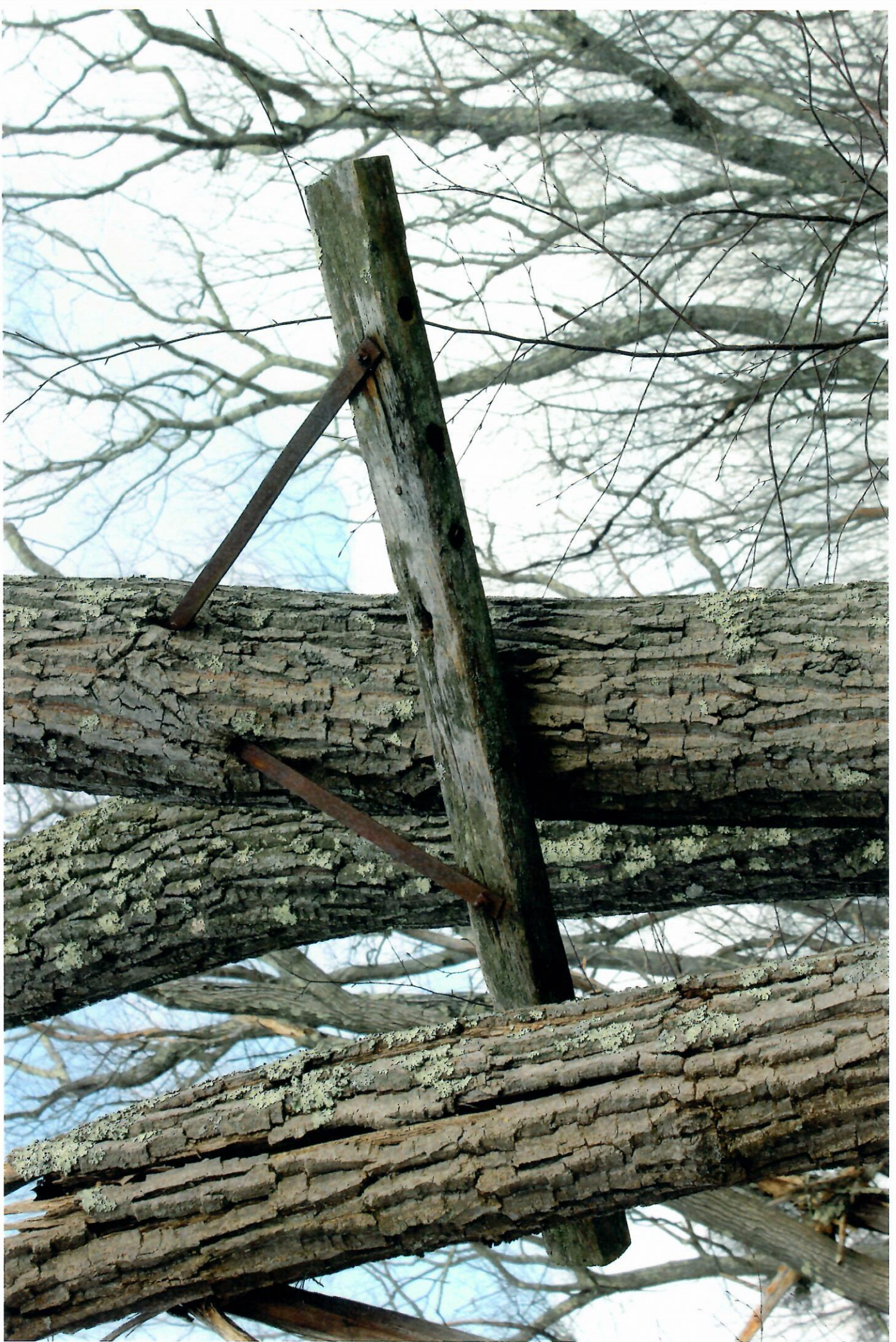
Cross anchor for one end of suspension bridge
